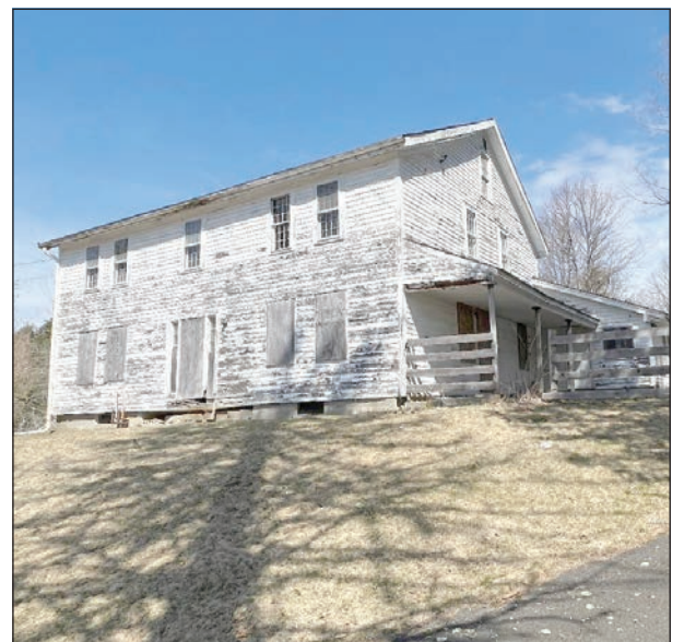
A decision to demolish Shepard Farm was made.
