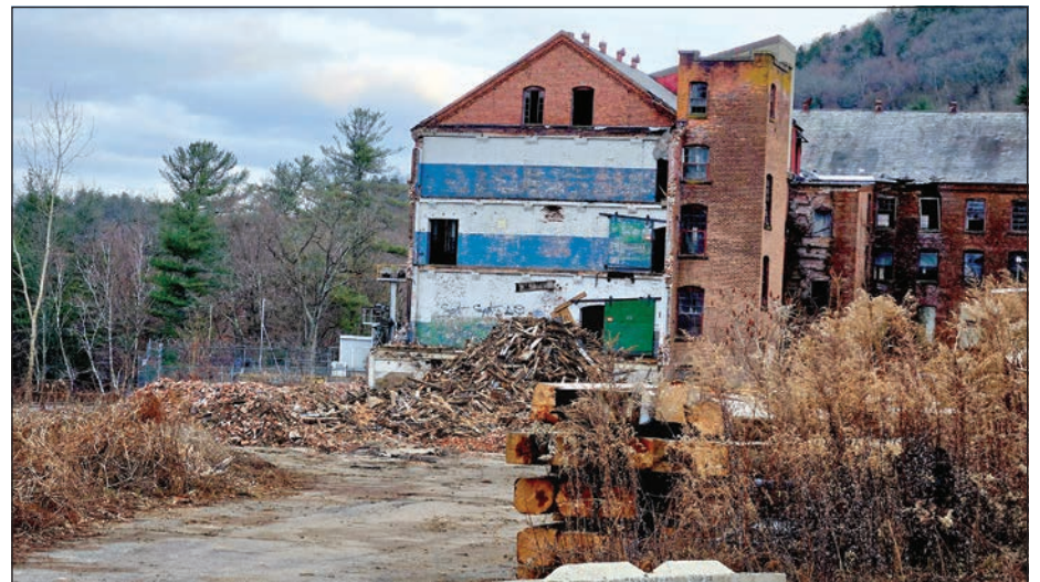
This shows the now demolished mill # 1 building.
