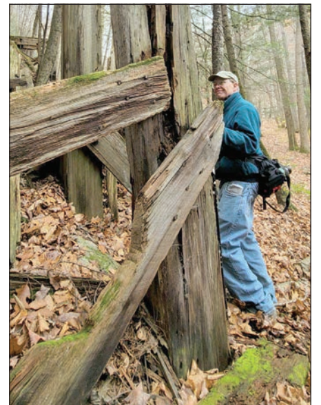
The Hikers explore this old wood structure.
