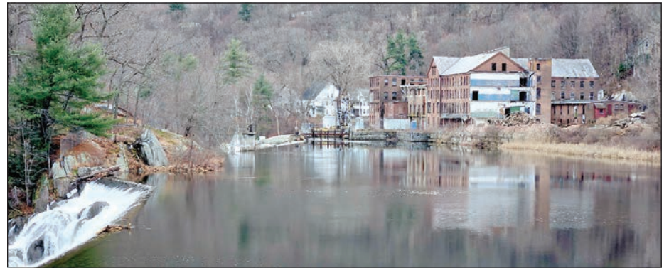
This photo shows vmill #1 from the river.
