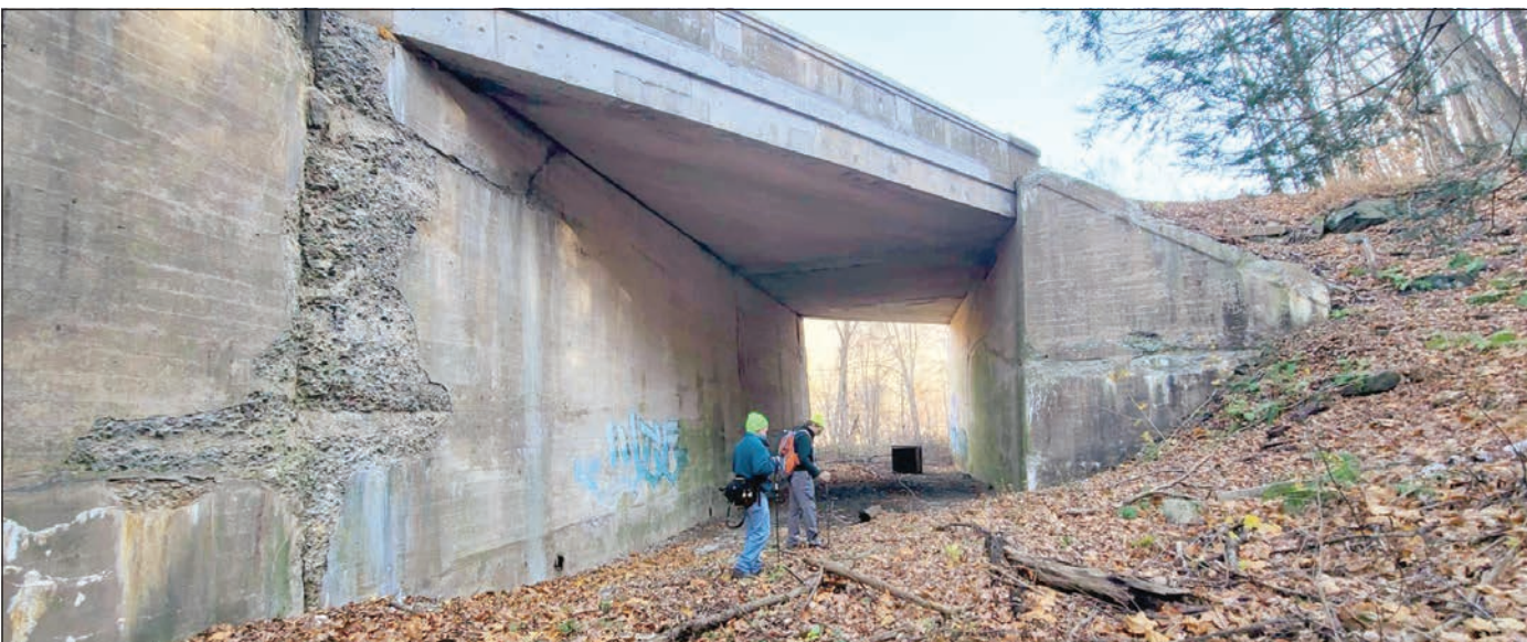
This photo shows the other end of the box culvert under Route 20.
