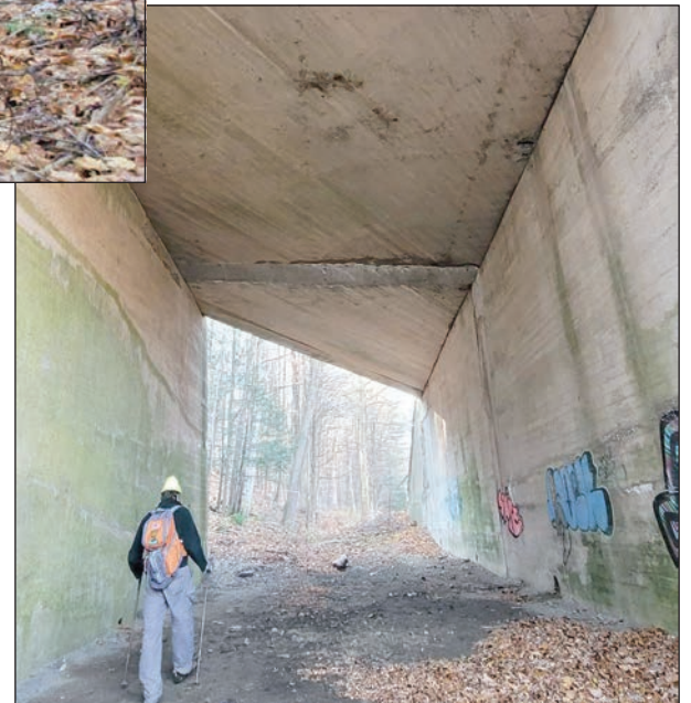
This is a view of the box culvert under Route 20.
