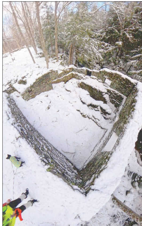
This is an aerial view of the saw mill foundations.
