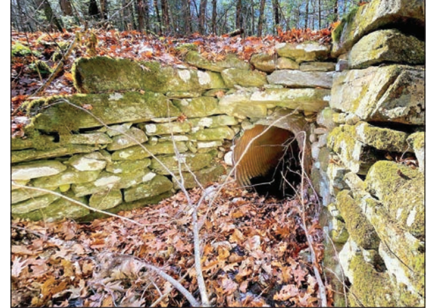
This stone laid culvert on the trail was built by the Civilian Conservation Corps during the Great Depression for the road to the pond.
