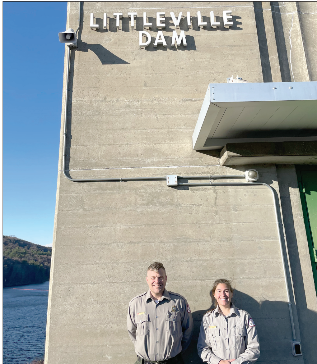
Interim Project Manager Keith Goulet and Park Ranger Marrison Eisnor, who work for the U.S. Army Corps of Engineers at Littleville Dam and Knightville Dam, both in Huntington, stand by the Littleville Dam. Turley photo by Wendy Long
