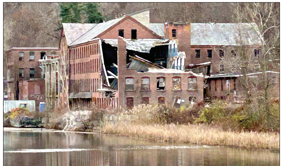
Remains of Strathmore Mill #1 is shown on Nov. 11 from the millpond.
