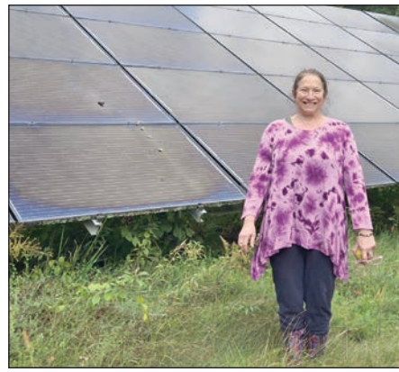
Ground mounted solar panels are another way besides roof mounted ones.
