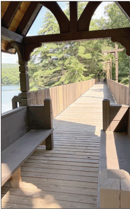
This is a view of Lake Pleasant through the bridge.
