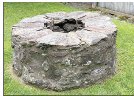
The well is located behind the Mission House.
