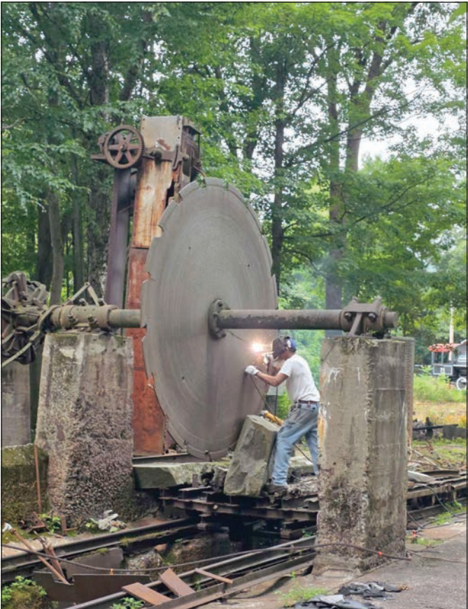
John Marcoulier welds the saw blade at the Chester Granite and Polishing Works in Chester on Thursday, Aug. 27.
