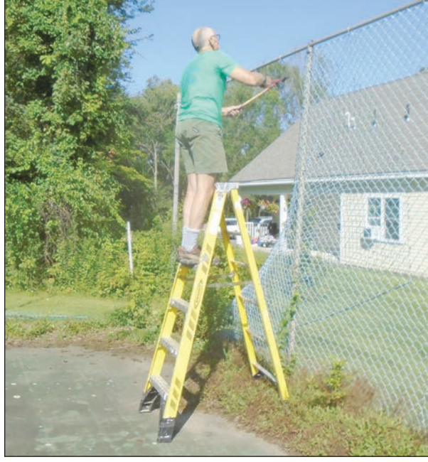
Michel Fairchild uses bolt cutters to cut heavy gage wire attached to the chain link fence.
