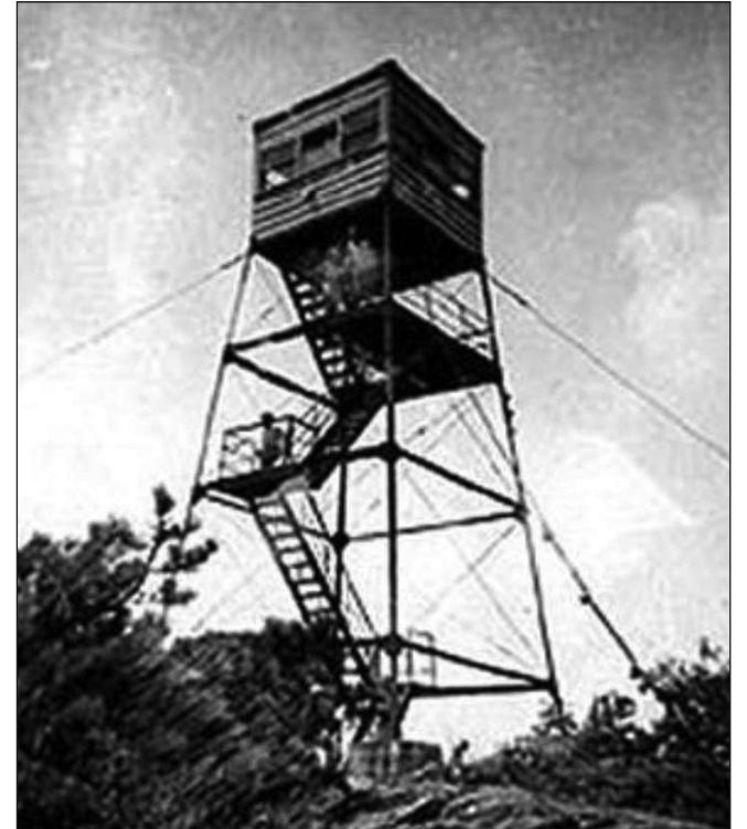
The original fire tower that was on Mount Everett.
