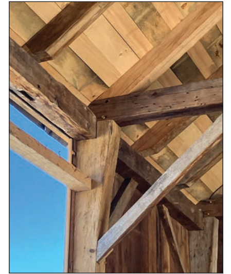
This photo shows the interior restoration work of the 1780 English barn.
