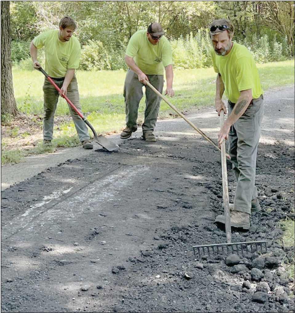
Turley Publications photo by Mary Kronholm Highway Department personnel, from left, Ryan Keach, Clayton LaPointe and Michael Carr prep Watson Park Road for paving project. Superintendent Ray Hultay expects the road to be paved before winter. The road will be level and safer for pedestrians as well as vehicular traffic.
