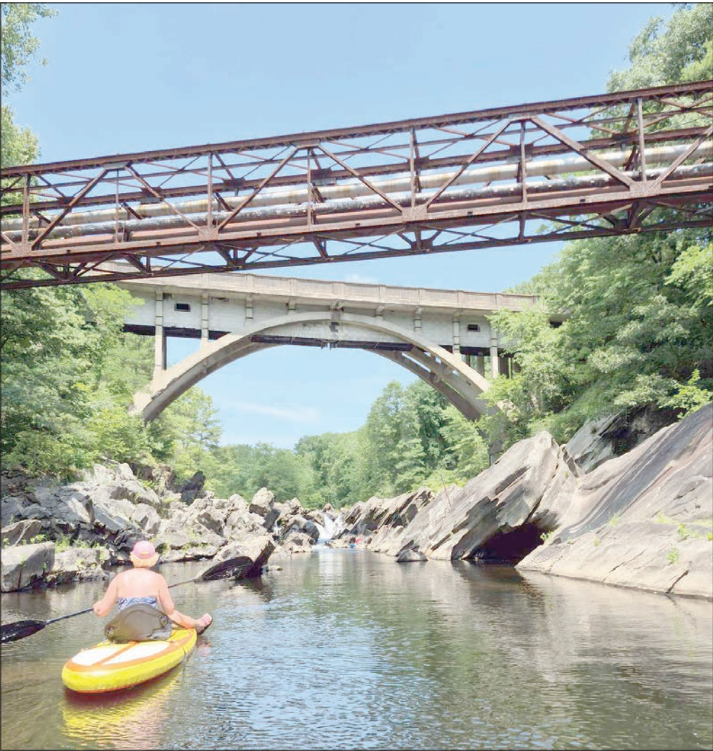
A member of the Western Massachusetts Hilltown Hikers approaches the potholes under the old Strathmore Bridge in the Woronoco section of Russell.
