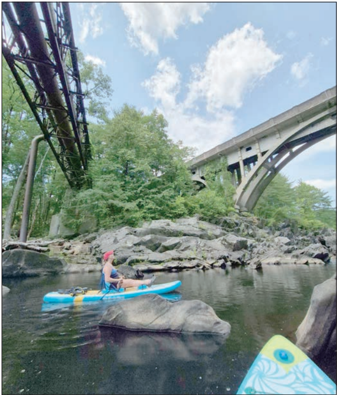
The potholes are under the old Strathmore Bridge, a favorite paddling location on the Westfield River.
