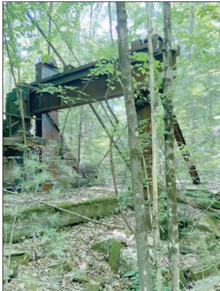
The frame, which held the granite saw, still stands
