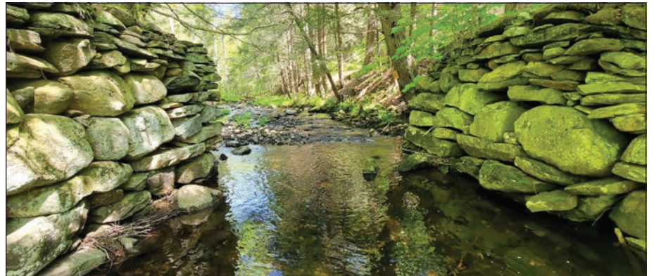
The stone abutments still stand for the old bridge from Middlefield to Washington.
