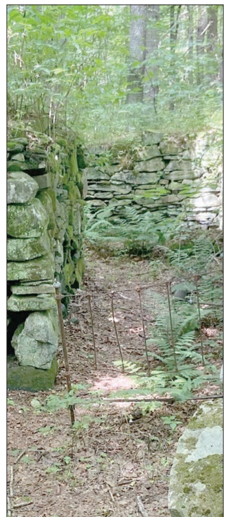
Remains of an early foundation on the Clam River Trail.
