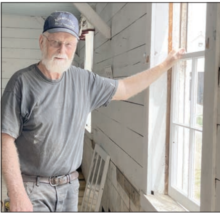
Rick Barnard helps install the new windows in the Agricultural Hall.
