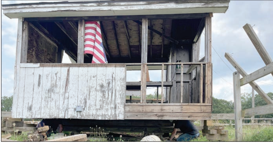
Horse show commentator booth is under restoration including leveling. Turley photos by Mary Kronholm
