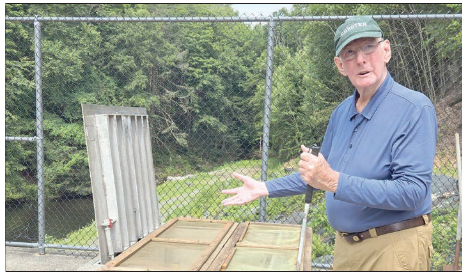
The town has received a $230k grant to replace two of the three filtration systems with new sand. The filtration is currently 20 inches below what it should be.
