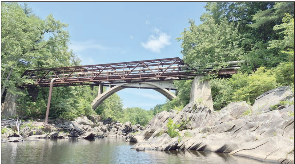
The old bridge to Strathmore Mill crosses the Westfield River.
