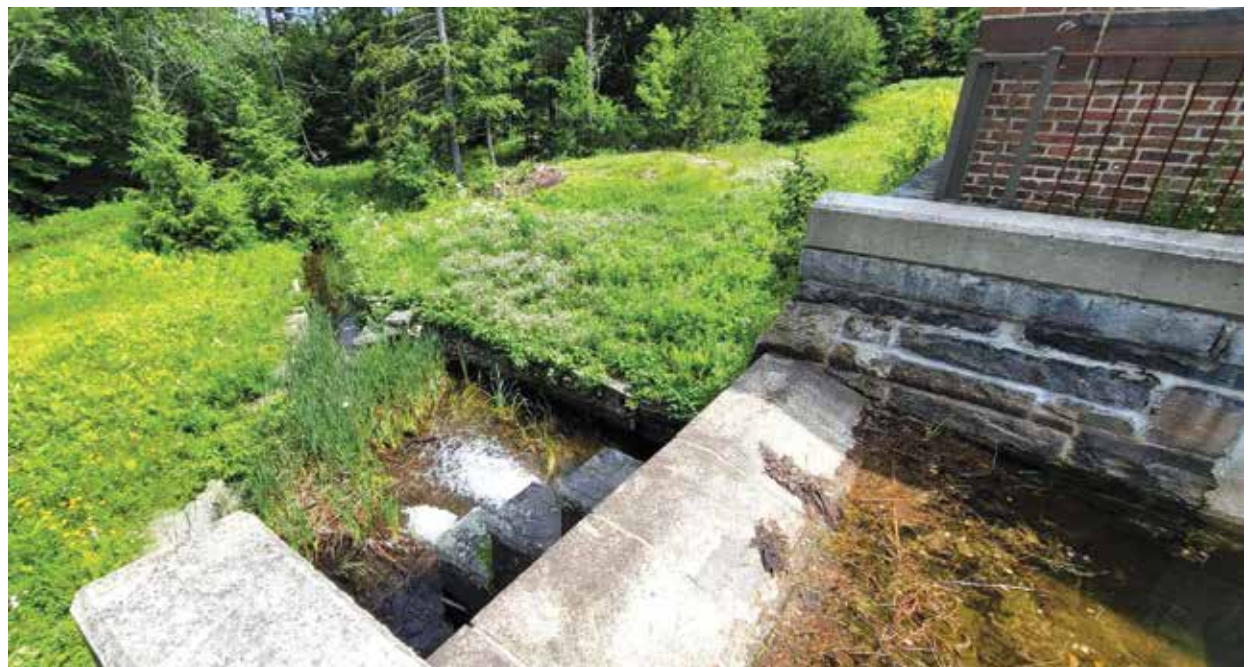
Here is a view of a stone spillway at the dam.
