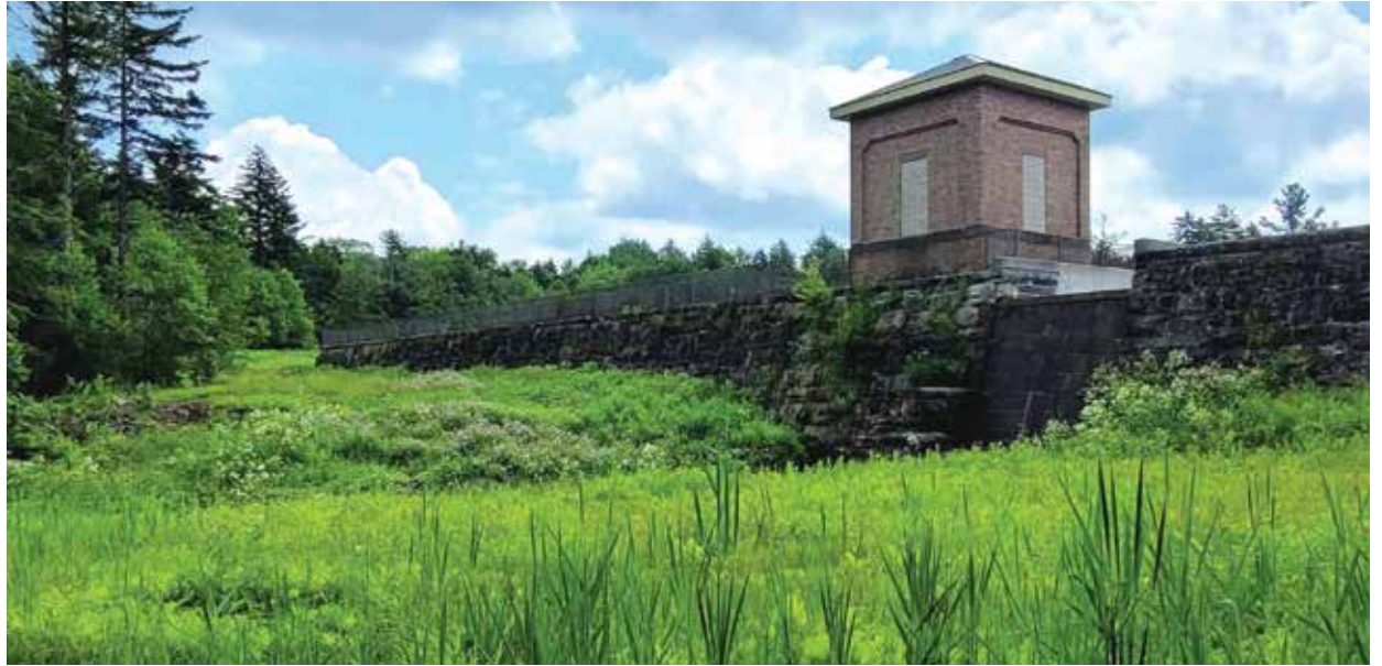
This is a view of the dam at Ashley Lake.
