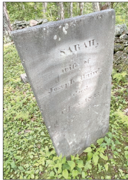
A headstone in Round Hill Cemetery shows wire brush damage.
