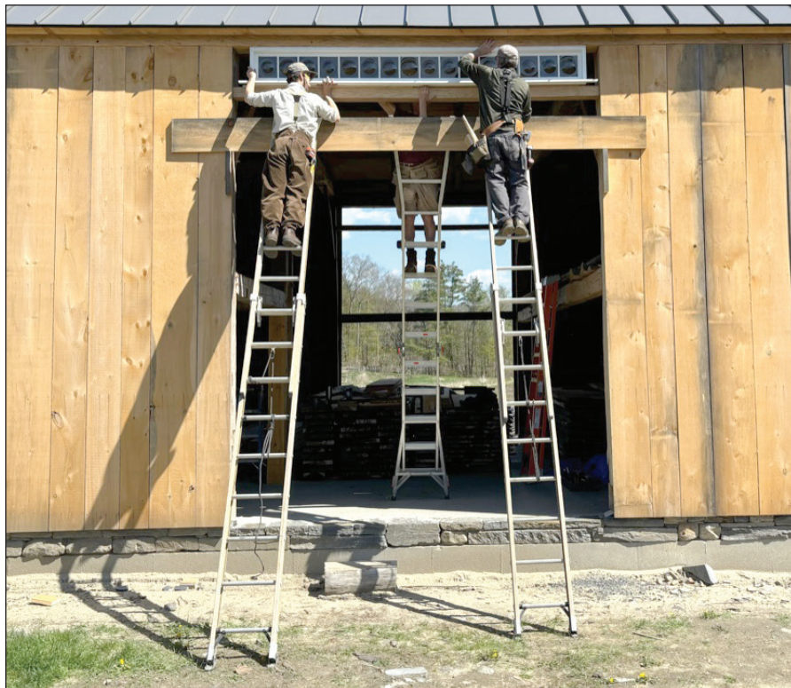
The Wilder Homestead and barn along with the Buckland Historical Society Museum will hold an open house and barn reconstruction on Sunday, July 14 from 2-4 p.m. Worker s fit the transoms to the 1780 barn. Submitted photo
