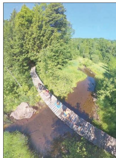
This foot bridges crosses the swampy area in Tyringham.
