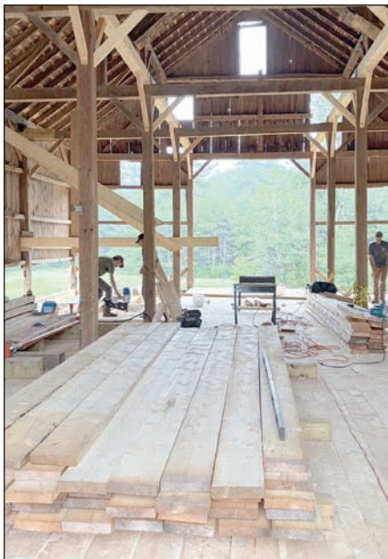
This photo shows the stacked lumber being used to complete the job.
