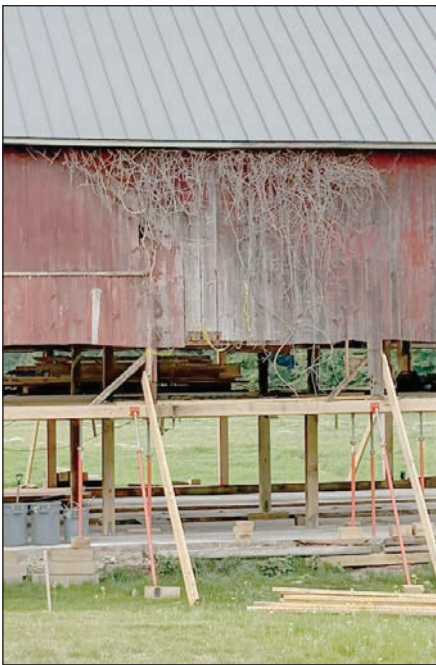
Here is another view of the barn.
