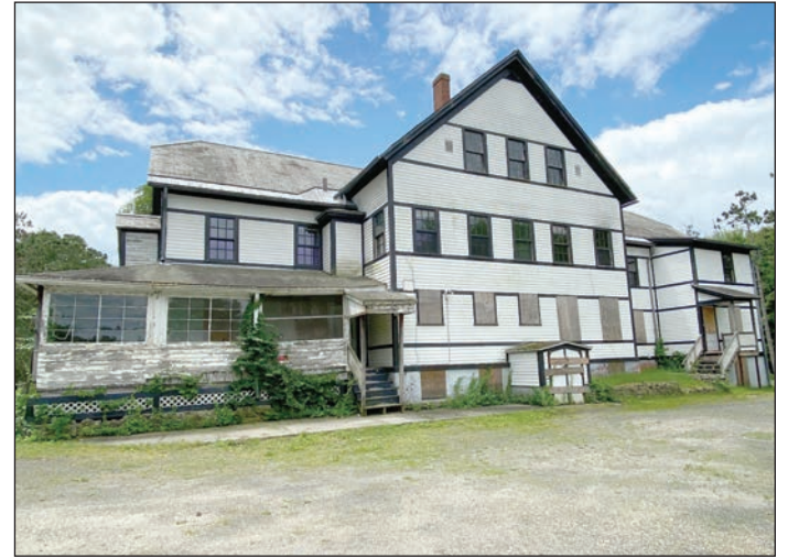
This shows a view from the rear of the house.
