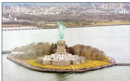
Liberty Island today with the statue on its pedestal and 11 pointed wall of Fort Wood that forms its base.
