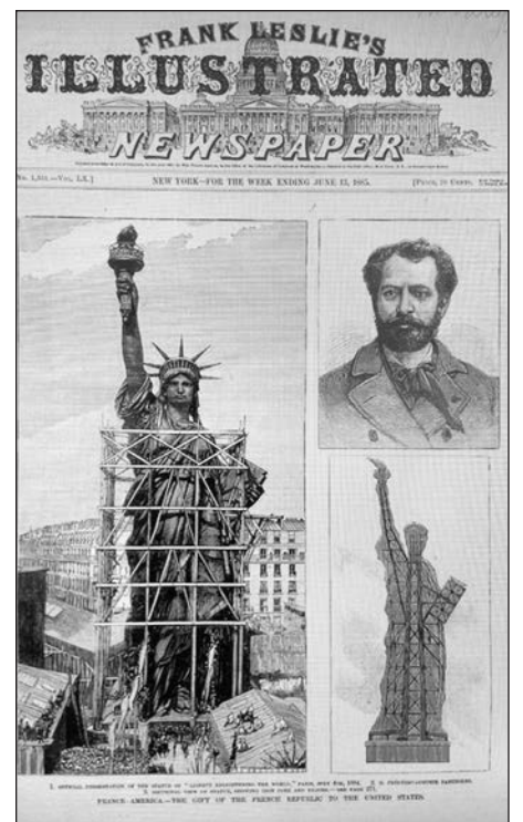
This publication shows the completed statue with scaffolding around Liberty, portrait of Bartholdi and a cut out showing the statue's interior structure.
