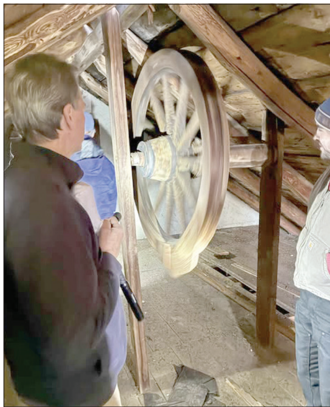
Visiting timber framer examines hoist wheel in attic.
