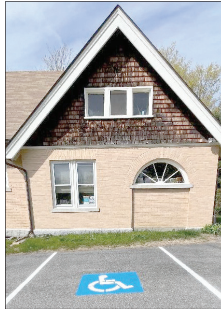
The library handicapped space moved closer to the entrance.
