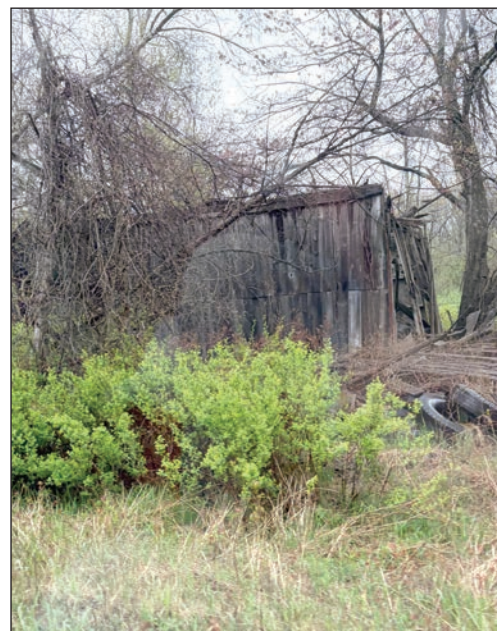
This is another view of the side of the collapsing barn.
