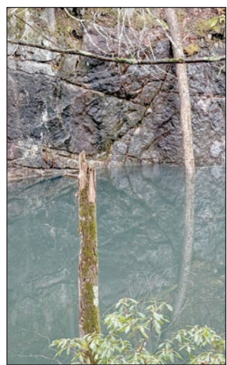
Turley photo by Deborah Daniels The large quarry site in Middleborough is now filled with water.
