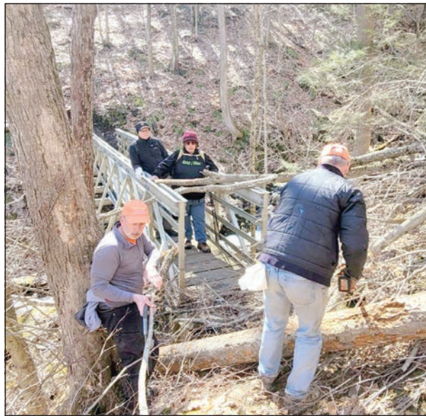
Tree work and trail repair takes place at the pedestrian bridge.
