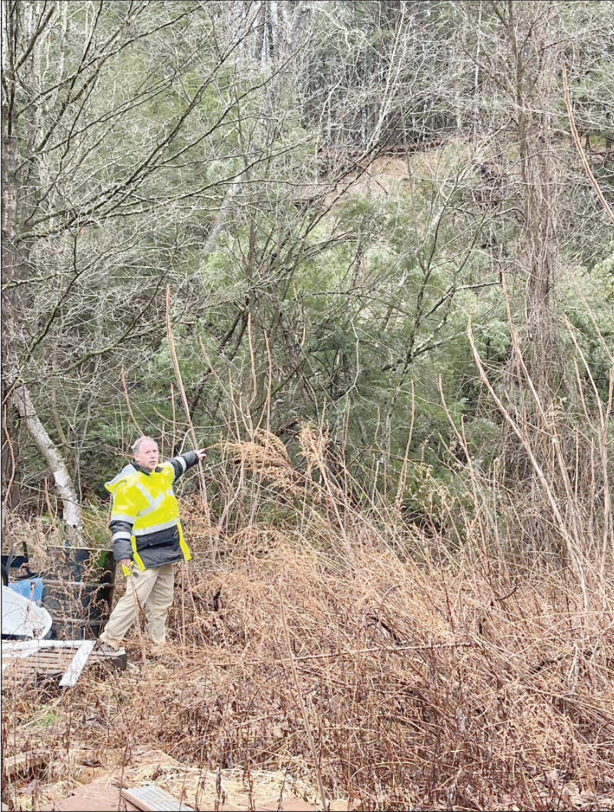
Blandford Highway Superintendent David Waldron points to the debris pile on Nye Brook Road from a land slide on March 28. Turley photo by Mary Kronholm
