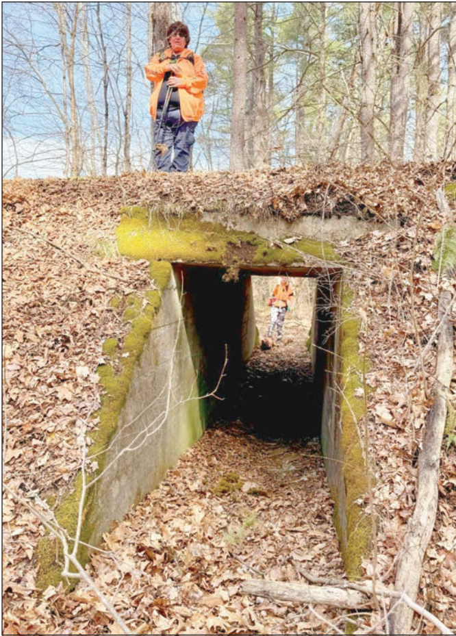
Above, Karen stands on a trolley railbed above a cattle crossing. These tunnels were created so that the animals in pastures could safely pass. Below, The 1910 Carnegie steel truss trolley bridge at the Wyantenuck Country Club.
