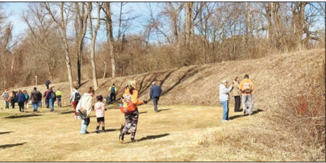
The raised hill on the Wyantenuck Country Club is the trolley bed. It was raised and lowered along the way to keep the grade manageable for the trolley cars.
