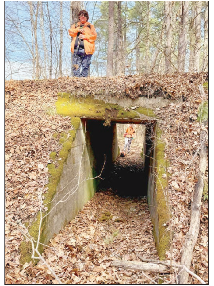
Above, Karen stands on a trolley railbed above a cattle crossing. These tunnels were created so that the animals in pastures could safely pass. Below, The 1910 Carnegie steel truss trolley bridge at the Wyantenuk Country Club.
