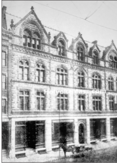
The Whiting Street granite building built by his estate in 1885, is located at 32 Main St. Holyoke. It was used by the paper industry and destroyed by fire in 1977.
