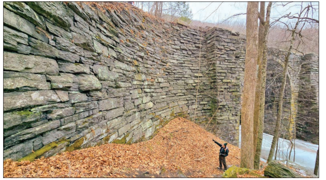
A Hilltown hiker points to the massive wing walls by the bridge providing prospective to the size of the arch bridge.
