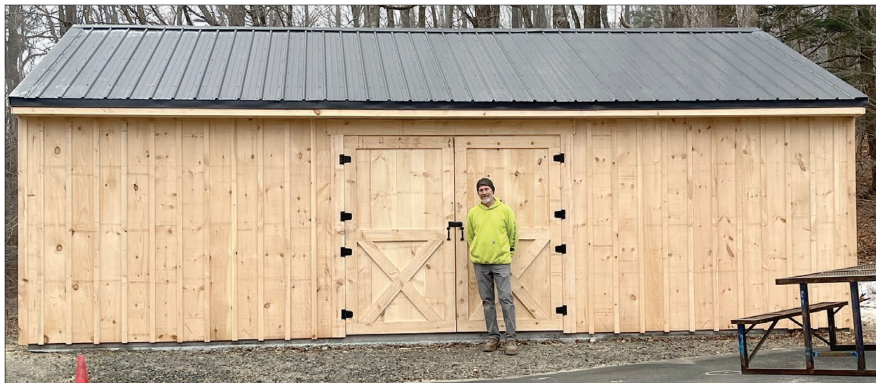
Bret Hartley stands in front of the “almost completed” Swap Shop building at the Blandford Transfer Station.
