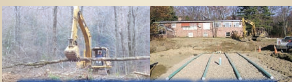
SEPTIC SYSTEMS DESIGNED & INSTALLED
