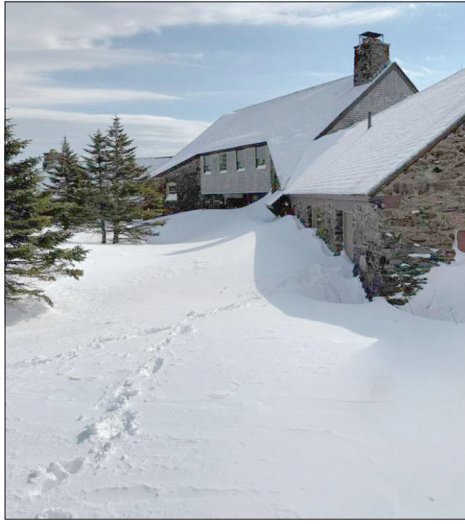
Bascom Lodge, located at the summit of Mount Greylock, was constructed between 1932 and 1938 and is a significant example of 1930s park architecture, named after John Bascom a DCR Commissioner.
