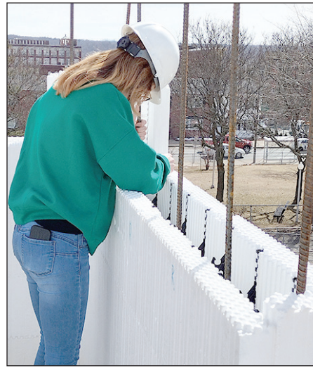
Dean student working with rebar.
