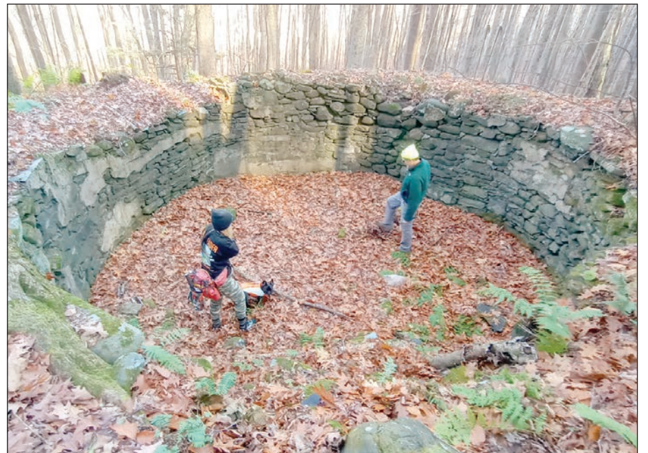
Two of the Hilltown Hikers explore the inside of what appears to be a cistern.
