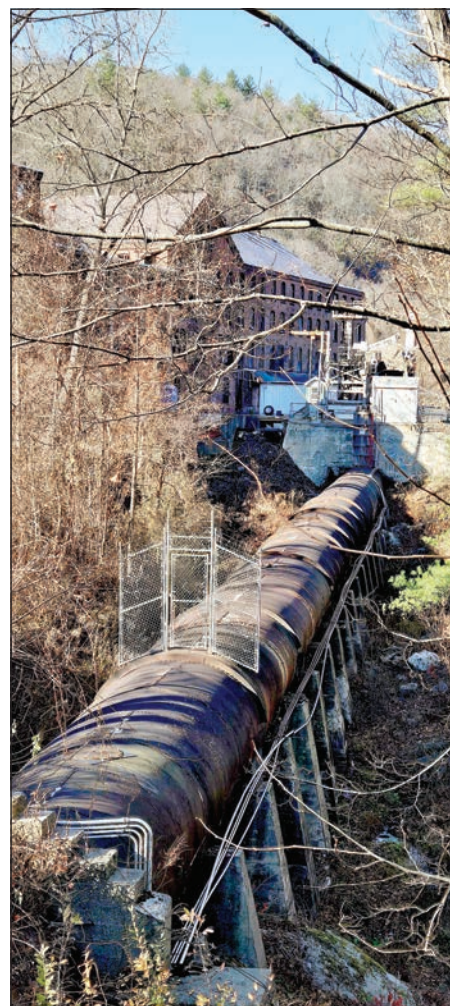
Strathmore Mill #1 is adjacent to a dam and hydroelectric power plant.
