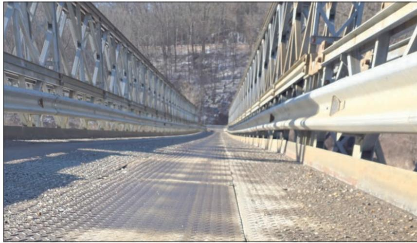
The deck of the Bailey Bridge, which was temporary when installed in the 1980s, has visible rust holes in the decking. It cannot bear the weight of most fire engines and the trucks needed in the demolition of Mill #2.
