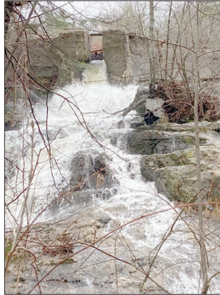
Stream water flows through a spillway in a pond dam. Photos by Deborah Daniels
