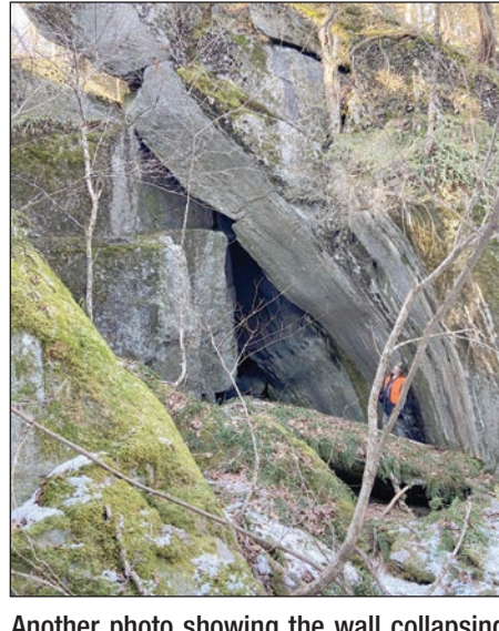
Another photo showing the wall collapsing down into a pothole with Hilltown Hiker Frank marveling at the site.
