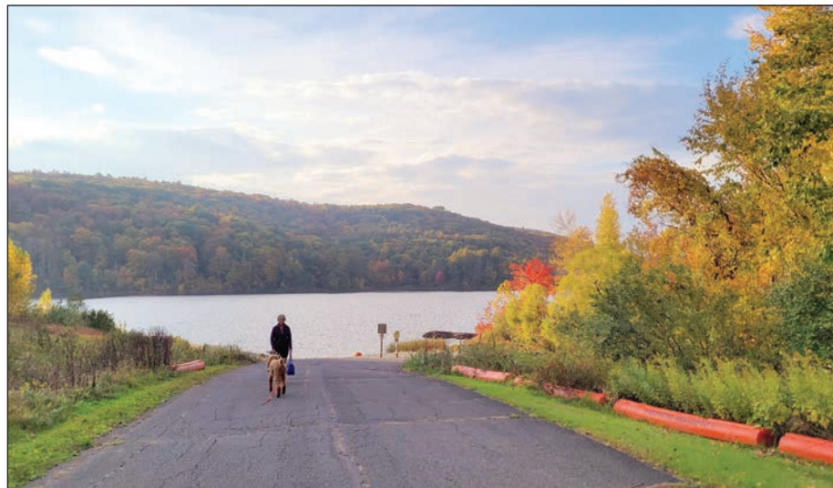
Littleville Lake has a large amount of parking at the southern and northern end. It was originally built with the idea of more recreation including swimming.
